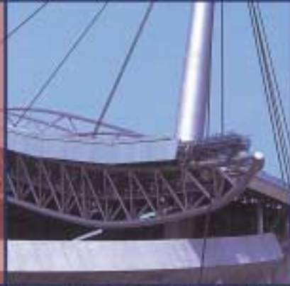
Hanging Roofs Structure
